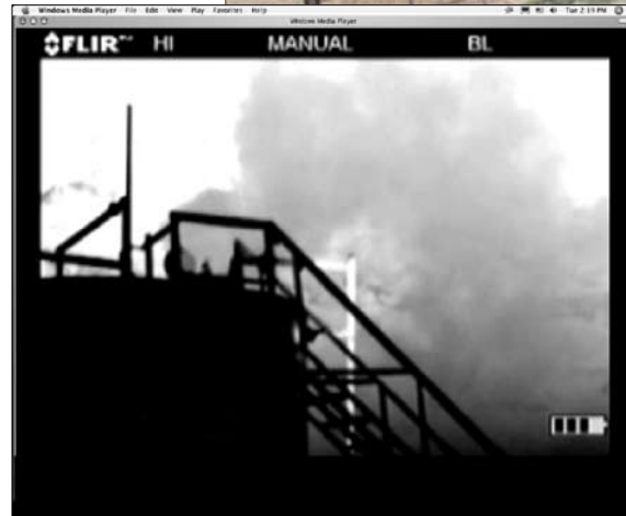
At left: Tank battery as seen with FLIR infrared camera showing a plume of natural gas billowing and sinking to the ground.
